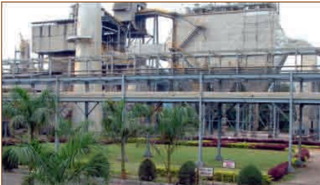
Captive Power Plant (CPP) located inside the unit at Jhagadia, Bharuch (Gujarat)
